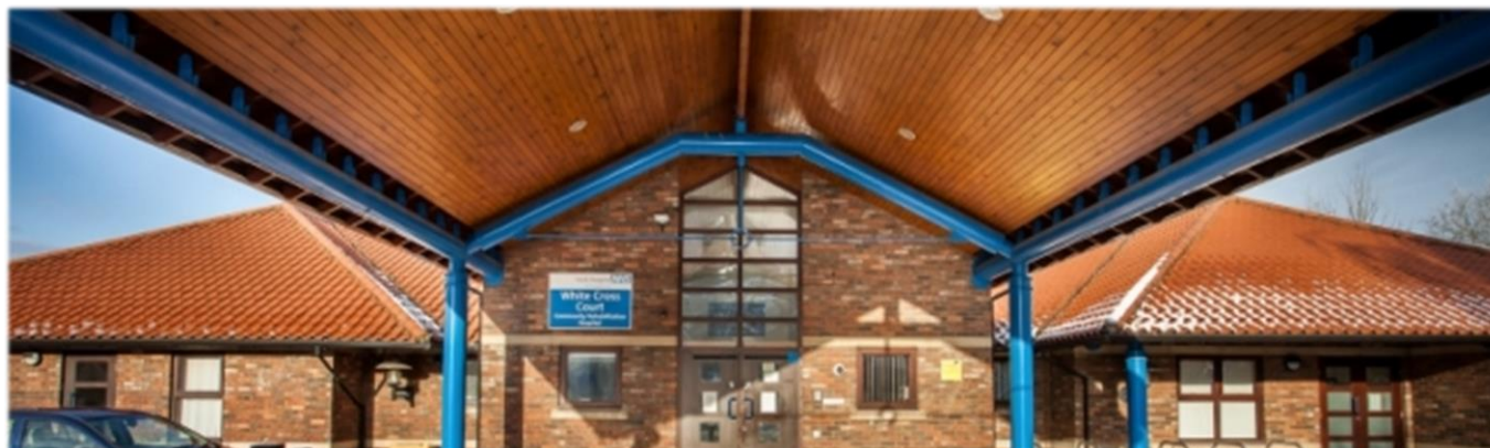
White Cross Court is one of our smaller sites and provides a range of rehabilitation services
