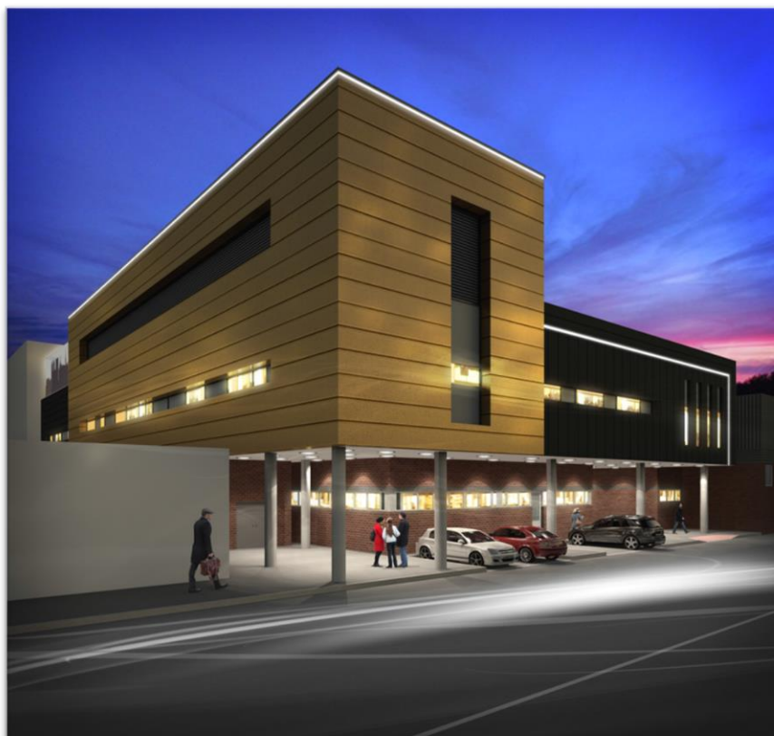
The new endoscopy unit, opened to patients in 2019, this modern unit has increased capacity and incorporates electrical submetering to measure energy use
